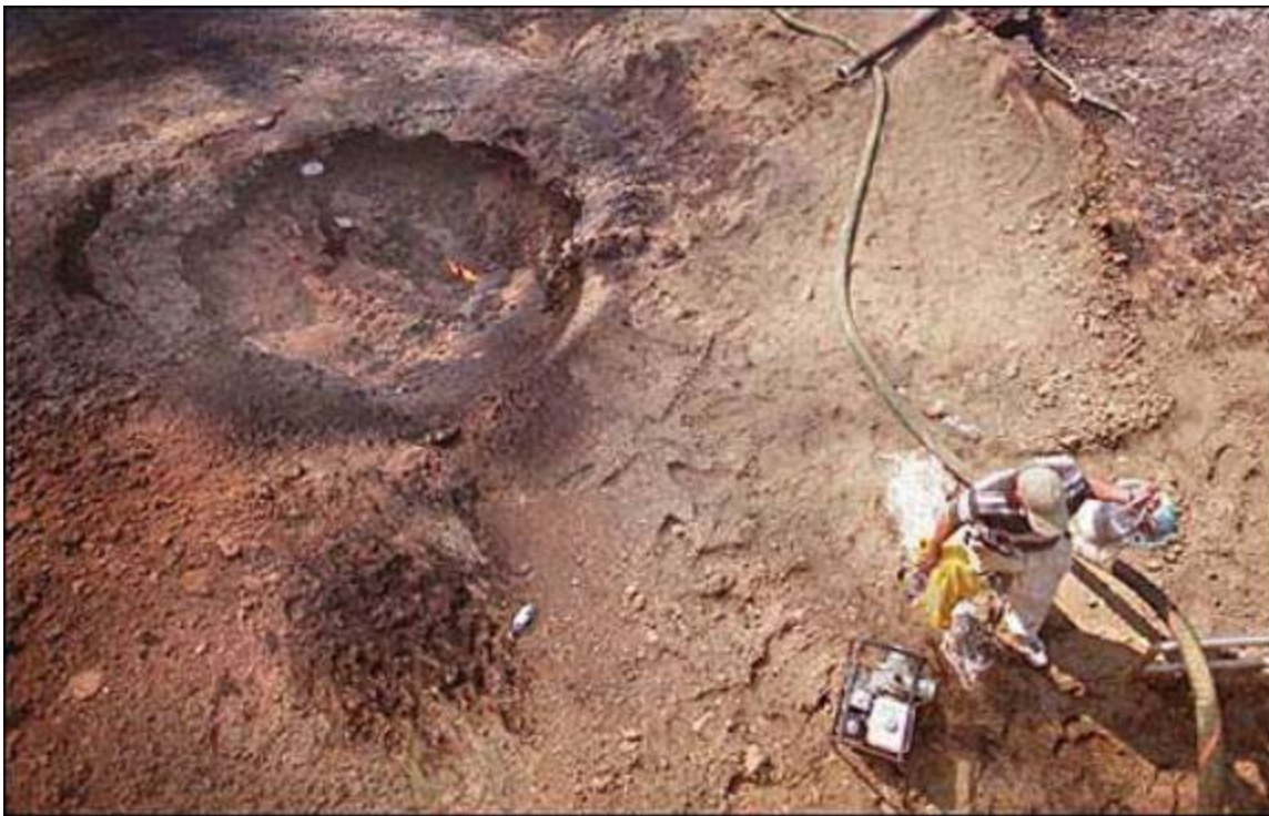
Figure 9-6. Larry Bateman, operations supervisor for the Bellingham Public Works Dept. walks past a crater near the water treatment plant Friday afternoon, June 11, 1999 (copyright June 11, 1999 Bellingham Herald , Reprinted with permission).
